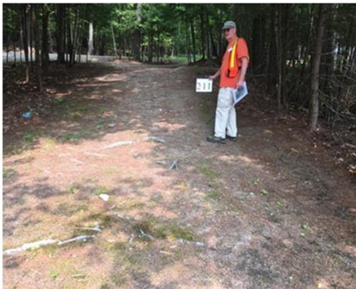
Figure 10. Runoff concentrates on these driveways then the eroded material washes into the lake
