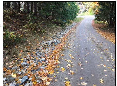
After photos of a stabilized by-pass channel (left) and stable ditches (right).
