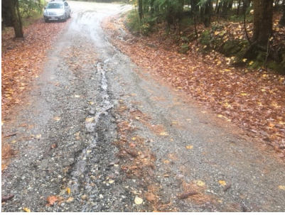
Before (top): Beaver Way's road surface was experiencing significant erosion due to poor surface material and insufficient crowning. Ditches were extremely unstable and eroding as well due to high runoff volumes.
