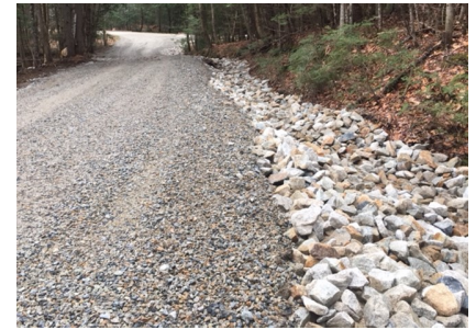
After (bottom): With new cross-culverts, turnouts and stabilized ditches, sediment is no longer carried to the stream tributary or the pond.
