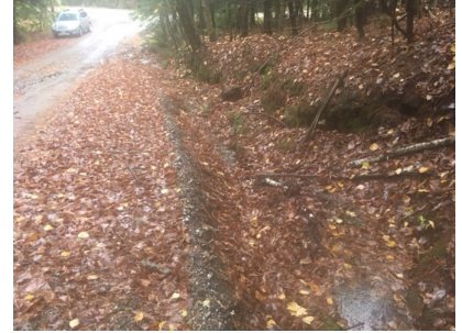
Before (top): Beaver Way's road surface was experiencing significant erosion due to poor surface material and insufficient crowning. Ditches were extremely unstable and eroding as well due to high runoff volumes.
