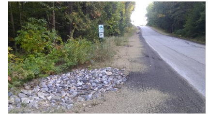
After (above): Shoulder stabilized with Reclaim and rip-rap.
