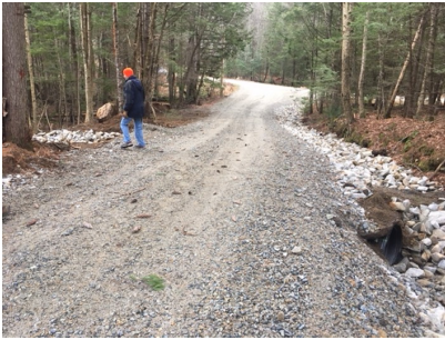
After (bottom): With new cross-culverts, turnouts and stabilized ditches, sediment is no longer carried to the stream tributary or the pond.
