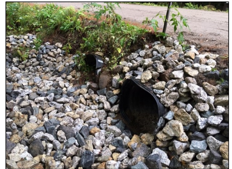
After (Right): Reshaped and rip-rap stabilized ditches and culvert inlet.
