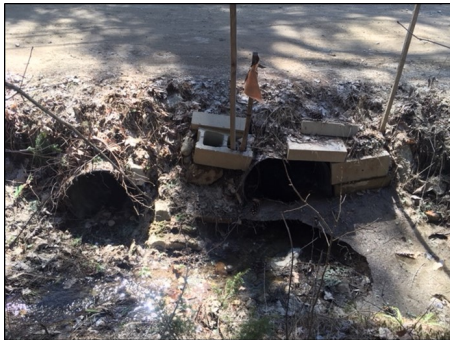
After (Right): Reshaped and rip-rap stabilized ditches and culvert inlet.
